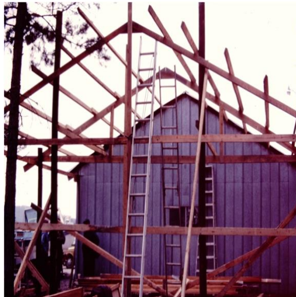
The photo above shows Joe's shop addition being built by the Oak Ridge Flyers (Courtesy of Charlie Hensley)
